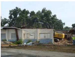
An old building was demolished in July...
