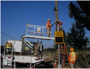
RMA staff installs radar vehicle speed feedback signs.
